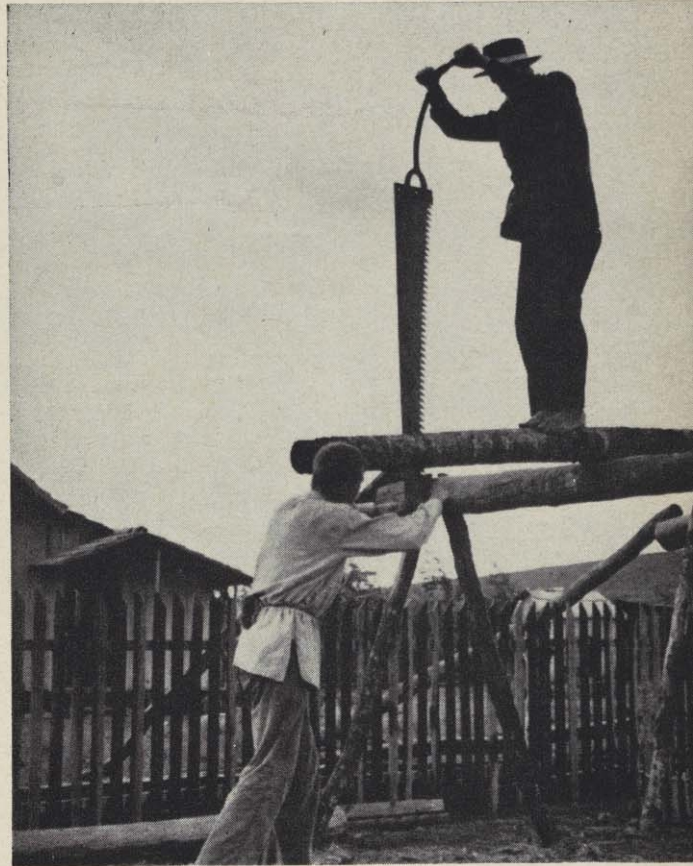
Primitive but effective, this method of sawing boards has seen much service in creating the numerous buildings completed in the four Old Believers' villages.
