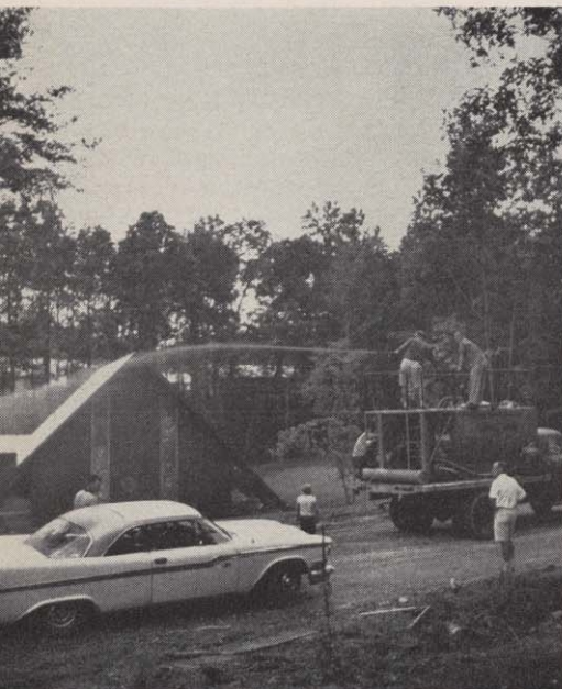
SEPTEMBER 10 —A volunteer detail of the congregation had raked and prepared the lawn. One member brought a highway tank truck which sprays seed, fertilizer, and lime, all in one application of a solution from a pressurized tank.
