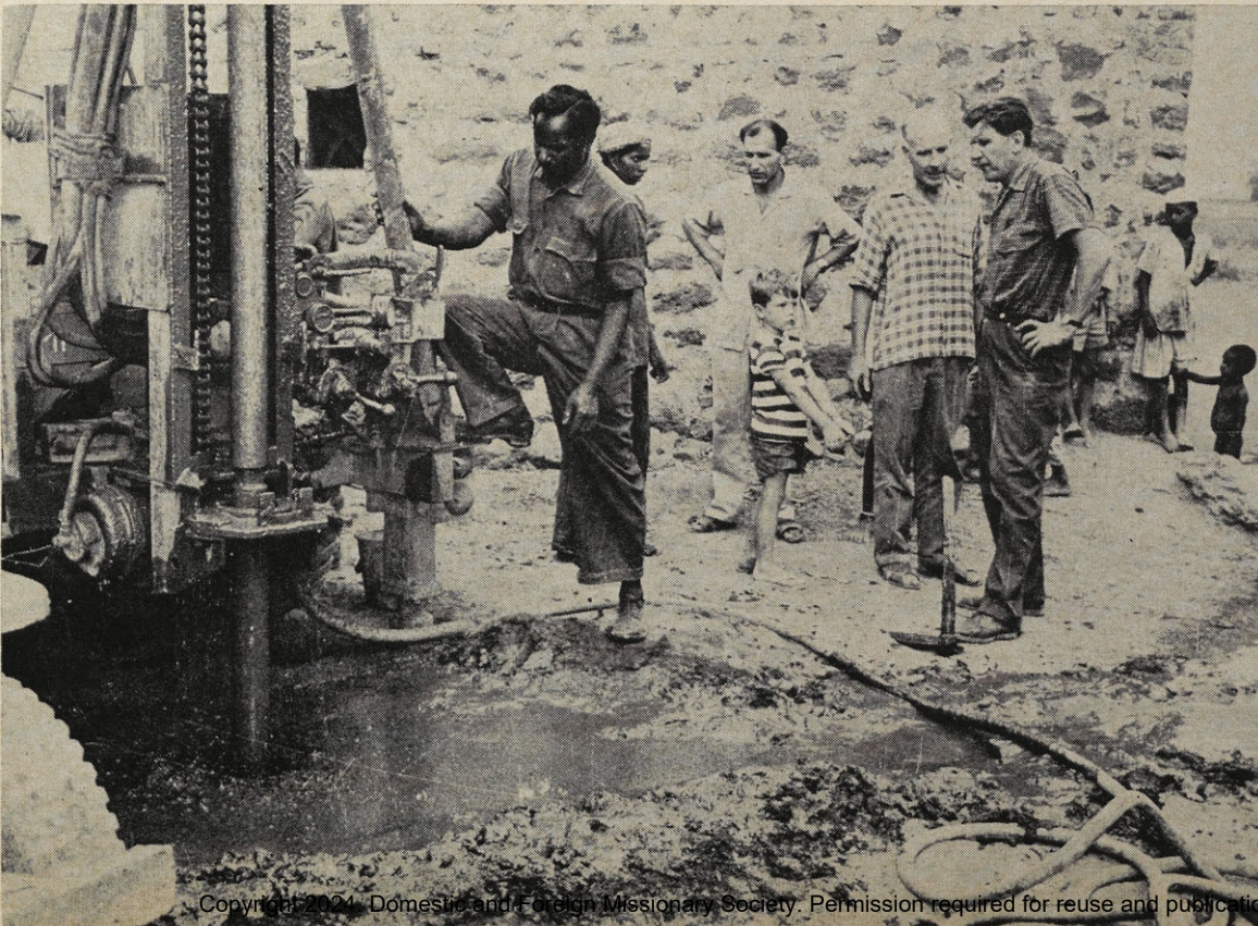
After earlier disappointment when a "strike" turned out to be a small pocket of water, a gush of mud heralds a strong supply, 170 feet below. Drilling one well takes a day.
