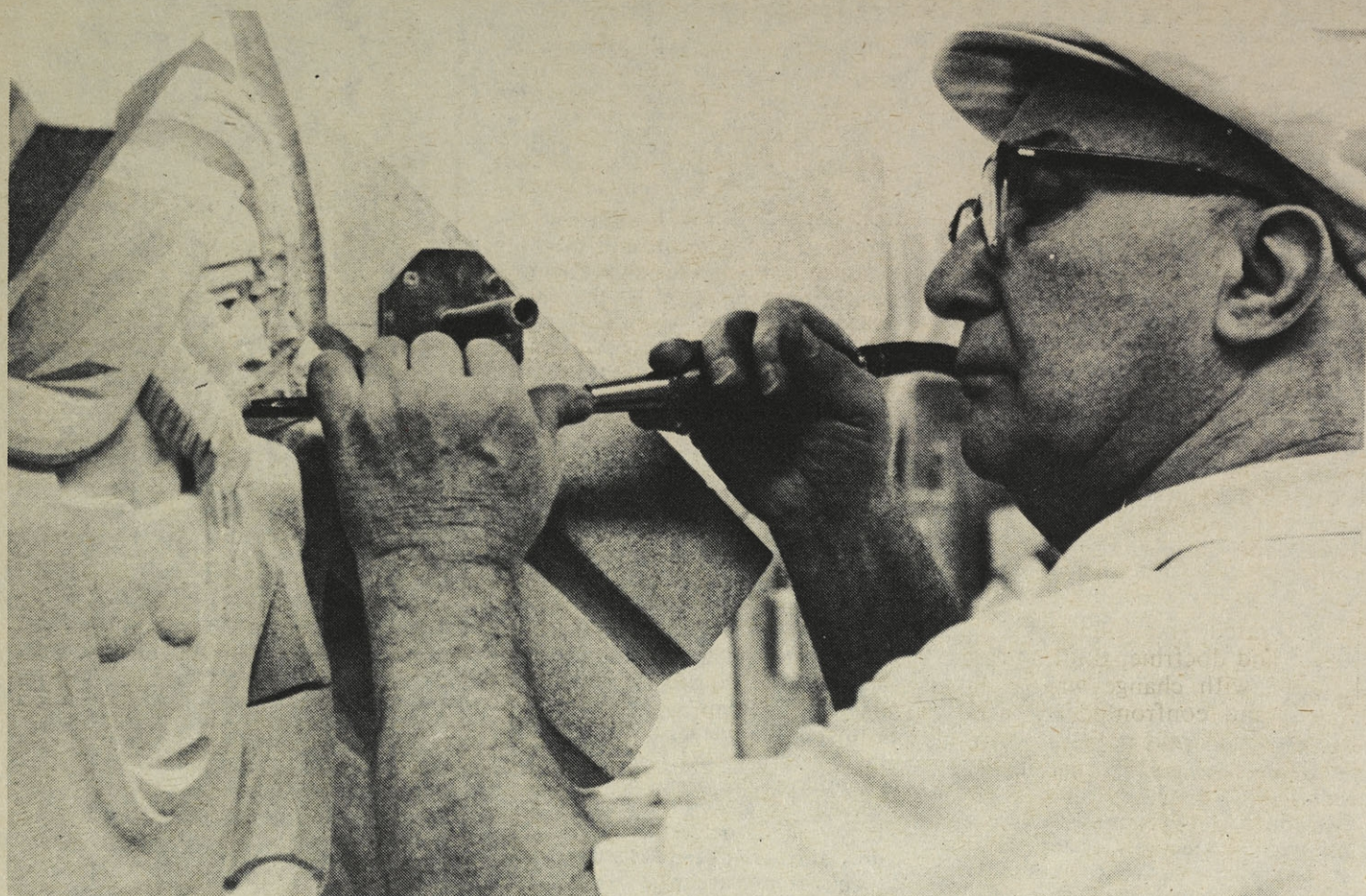
SCULPTING HISTORY INTO STONE , above, is helped by using an electric chisel, a new aid, but the stonecutter's art is an old one. The stonecutters' faces, below left, will eventually be placed beside those of traditional saints and martyrs, below right, atop Washington's Cathedral.
