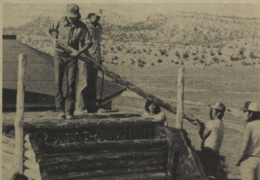
A LOG AND ADOBE solar heater is built by Indian trainees. The system includes a "collector" box which was later placed at the front slanted to catch the rays of the winter sun. Seven tons of rock store heat inside the log bin.
