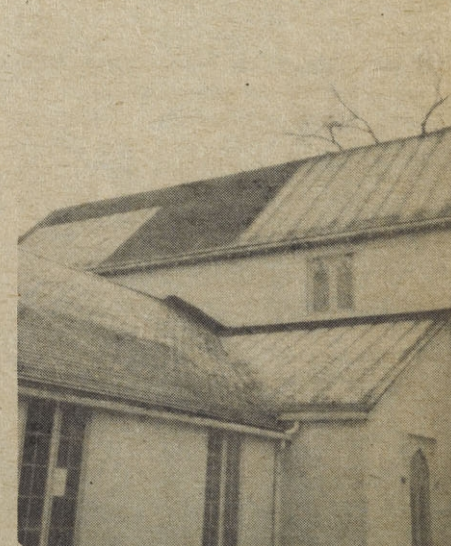
The roof tells the story of heat loss at St. Luke's, Chelsea, Mass. The uninsulated portions show clearly as black.
