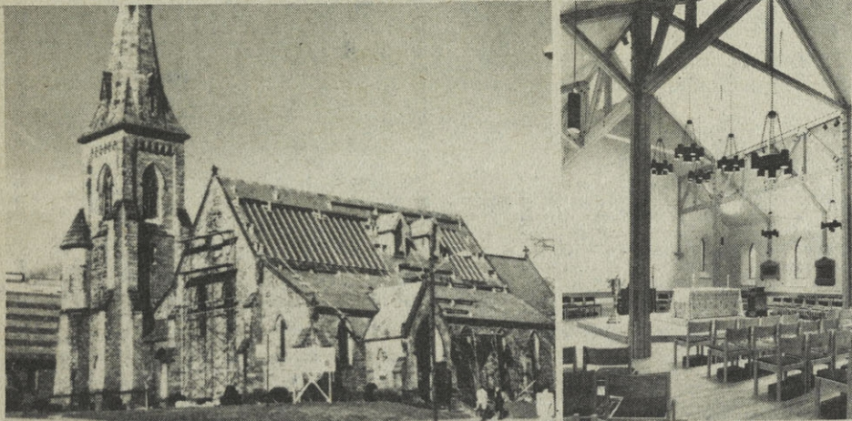
With a high, sloped roof and southern exposure, St. Paul's was ideally suited to the solar system which now provides half of the church's heating needs and has a gas-fired back-up furnace. Exterior renovations carefully followed Richard Upjohn's design lines.
