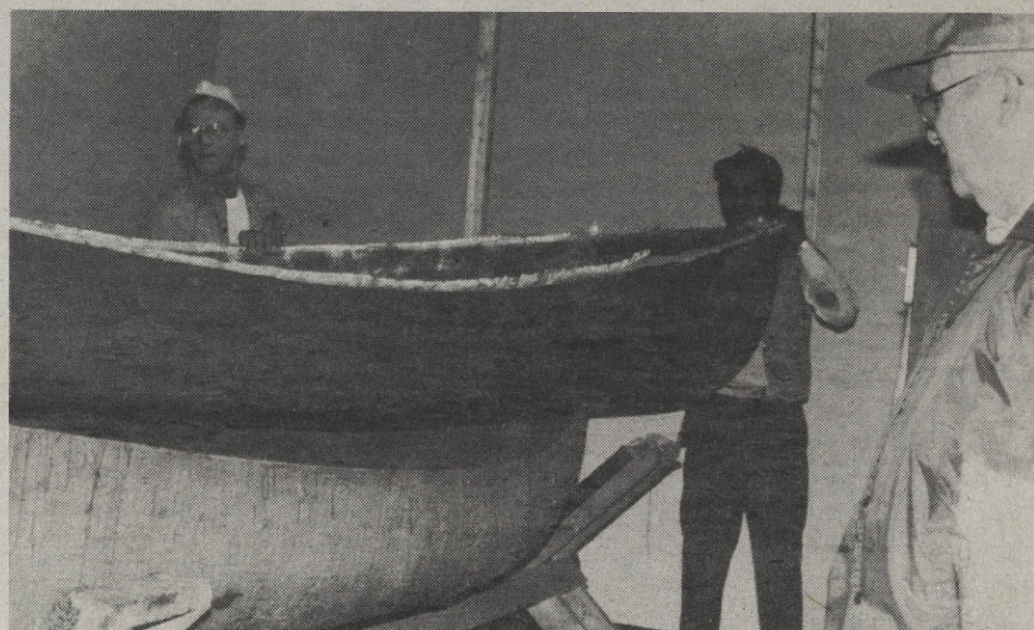
Color it purple. The canoe ordered by Presiding Bishop Edmond Browning is eased out of its mold at the Keystone Canoe Factory in West Virginia.
