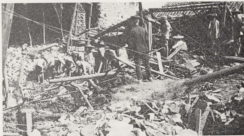
OUTSIDE BOONE COMPOUND three bombs caused this wreckage. Inside the compound, damage was limited to broken doors and windows. Workers are here clearing away debris in search of possible survivors
