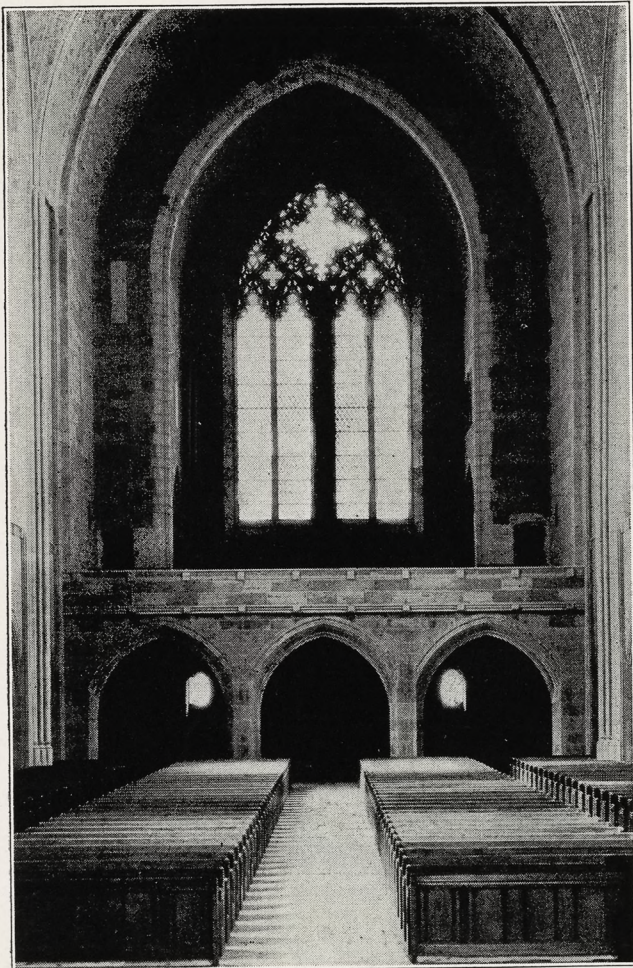
Looking toward the back of the church from the chancel, showing the great west window. The tile vault and side walls contain part of the acoustic installation, the work of R. Guastavino & Company
