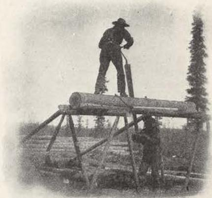
The primitive saw-mill where our lumber was manufactured
