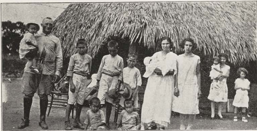
THATCH HUT USED FOR SERVICES IN CESPEDES
